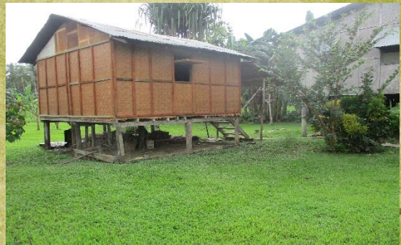
New walls for the kitchen
